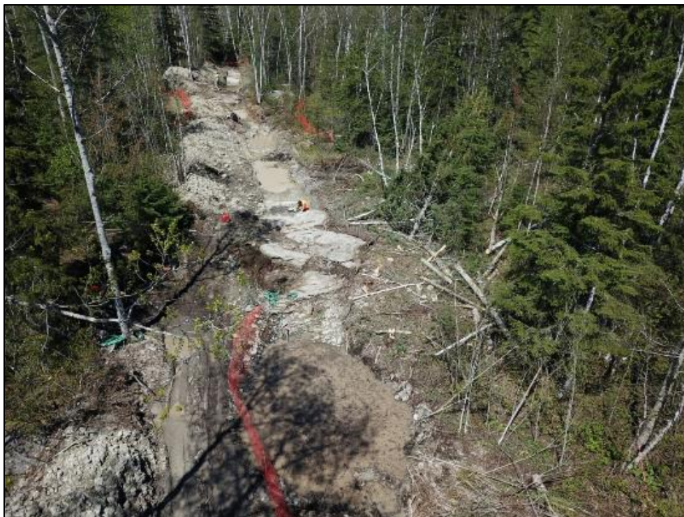
Figure 8-3 Trenches at Aukeko Site 2018
