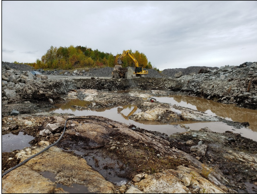
Figure 8-6 2019-2020 Stripping on Granada Property
