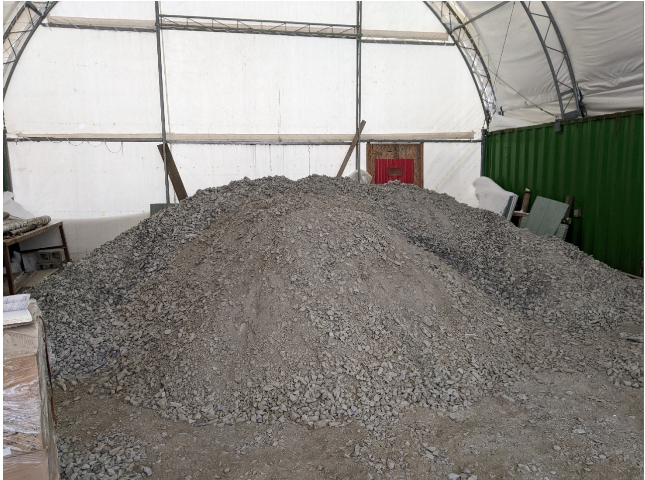
Figure 11-4 Bulk Material Stored in a Shelter
